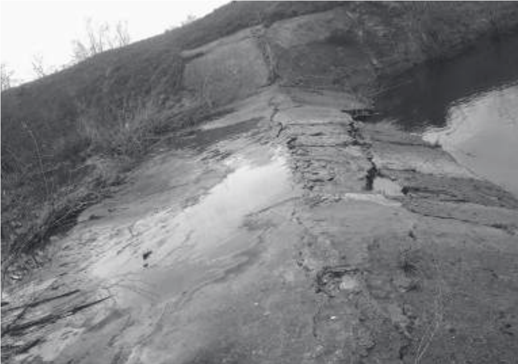
Fig. 2. View on the overflow dam
