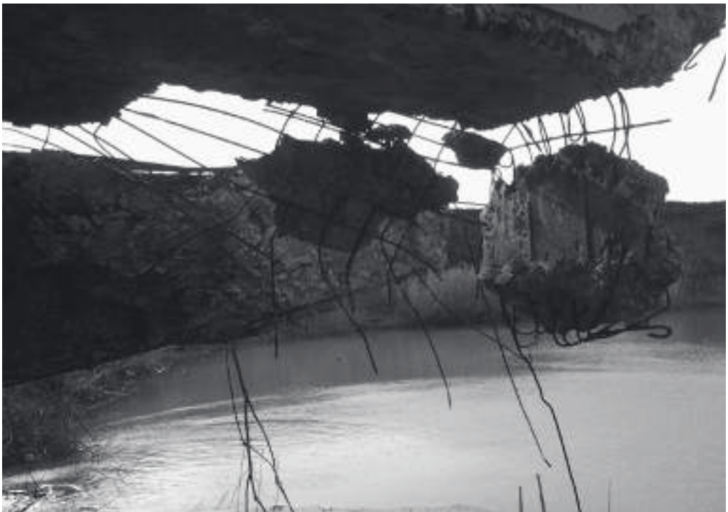
Fig. 1. View on the conjugation structure – the console spilling
